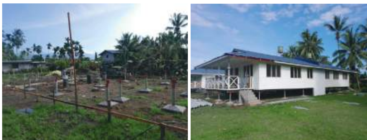
Picture courtesy of RPNGC PIP Team: Pictured is the construction and completion of five (5) duplexes at Bumbu Barracks in Lae, Morobe Province.
