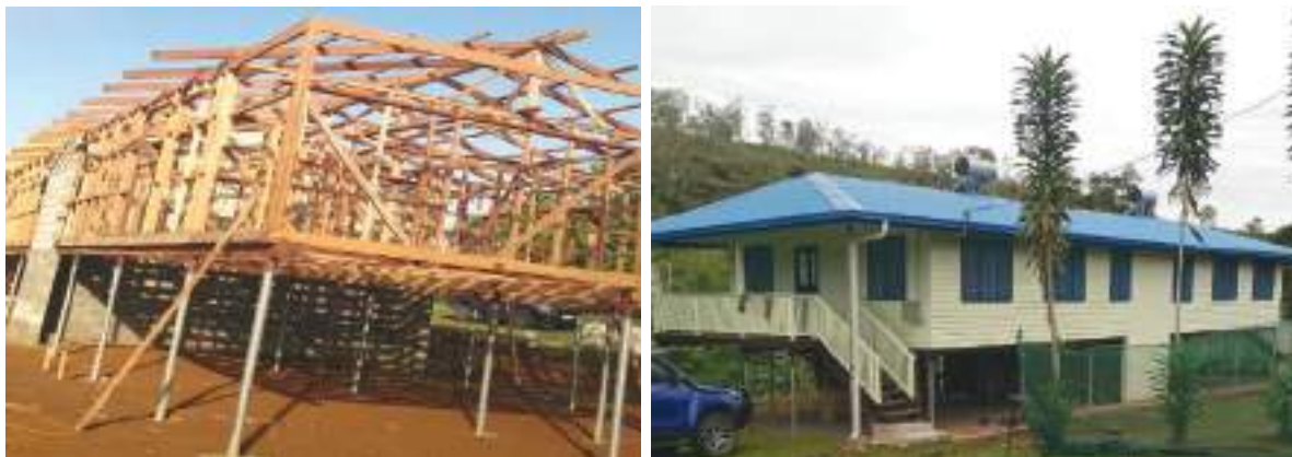
Photo courtesy of RPNGC PIP Team: One of five duplexes built at Sogeri Police Barracks, Central Province. Left: during construction; right: completed structure.
